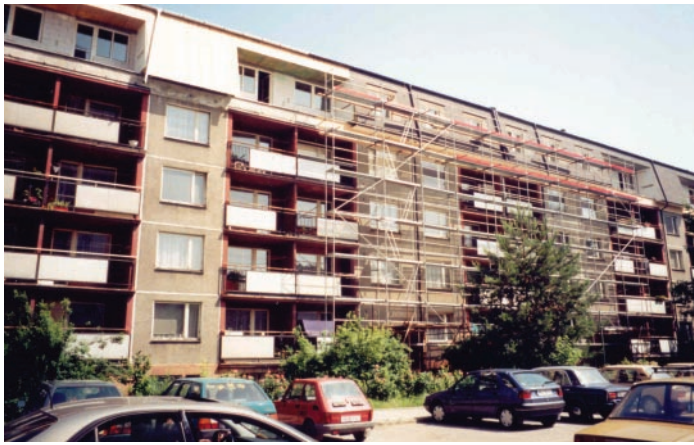
The project looked at innovative ways of increasing existing housing stock, such as this method used in Prerov. The municipality added an additional floor of housing under the roof of existing buildings.
