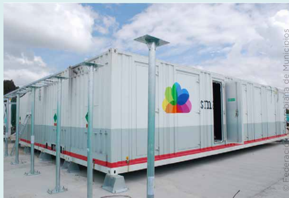
Smart Cloud data centre
