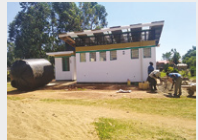
Toilet facilities being constructed in the Butere Ecopark, Kakamega County
