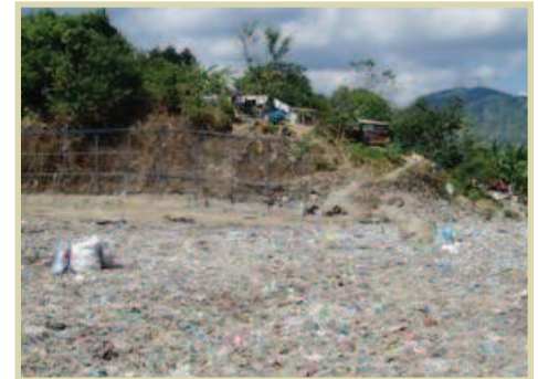
Newly erected litter fence at Olongapo landfill
