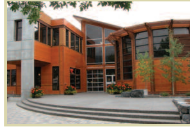
FCM supported Canmore, Alberta’s feasibility study for greening its Civic Administration Building with a $34,250 GMF grant.
