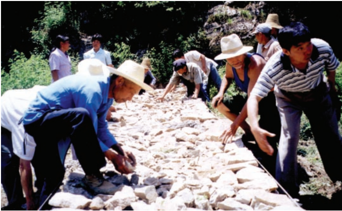
Construction of erosion control structure by villagers, farmers, and local authorities.
